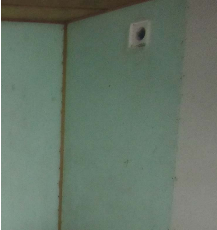
Ventilation intake plugged with a rag
